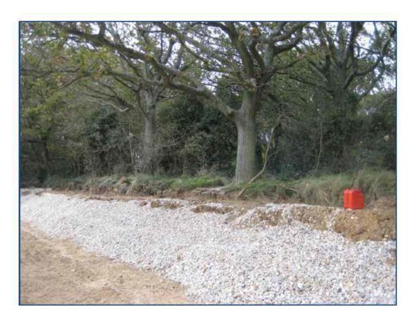
The shingle layer over the earth bank helped, but the slope would need cladding in Armorloc blocks as a long term solution
