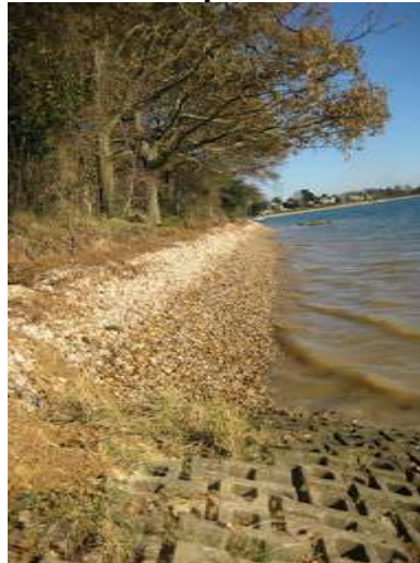
2012 earth bund completed
